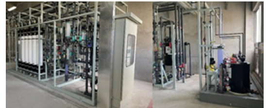
Cooling Tower Blow-down Recovery system
