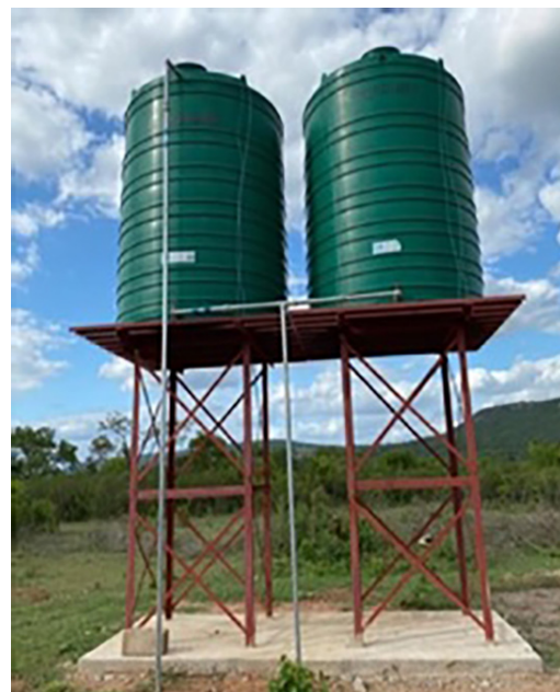
Construction of a well in Hhohho (Thandeka Ngobe/WaterAid Eswatini)
